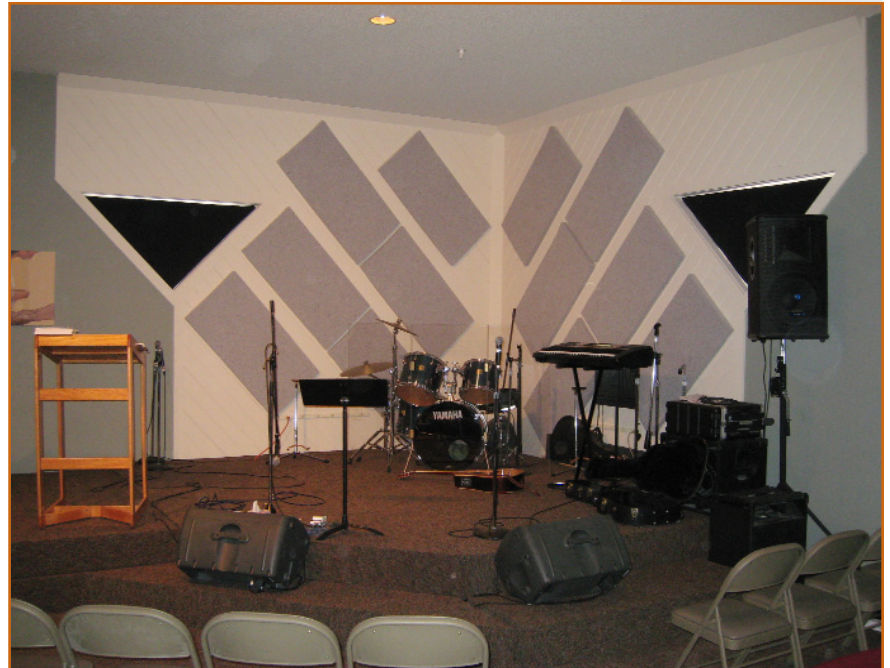
River Heights installed 12 (2' x 4') x 2" thick Echo Eliminator™ panels on the walls behind the stage. Thick panels were two inch. Used to reduce the amount of mid. & low frequencies created by the drums.
