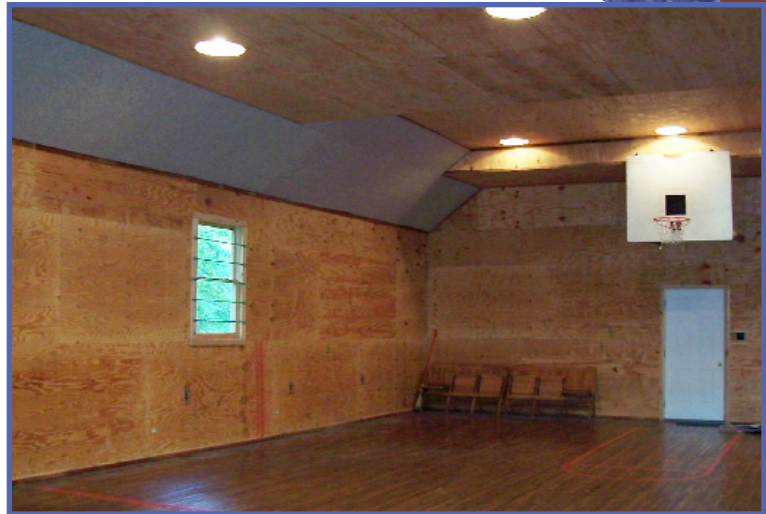
The acoustical panels were put on the angled part of the ceiling because the location was an even balance of ease of installation.
