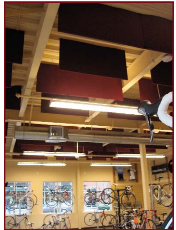
The owners and employees chose to install eighty of our 1" thick, #3 lb. density Burgundy Echo Eliminator panels as an economical yet effective and simple way to treat this space. The grommets were installed and the panels were installed by the employees. It is very important to keep the fire suppression sprinkler system in mind when considering hanging baffles.
